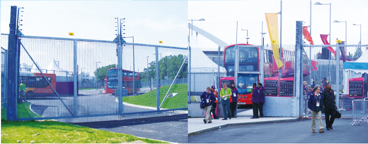
柵欄之架設。(Photo Credit: Sludge G, https://www.flickr.com/photos/sludgeulper/7644897068 , https://www.flickr.com/photos/sludgeulper/7721560134 )
